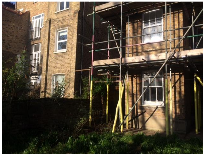
Rear view of the site towards the south side.
